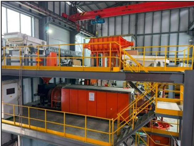
Figure 1: The newly installed intensive leach system.
