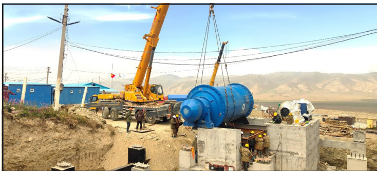
Figure 2 Installing the new ball mill.
