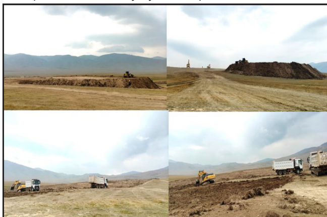
Figure 3 Excavation of the new tailings dam.
