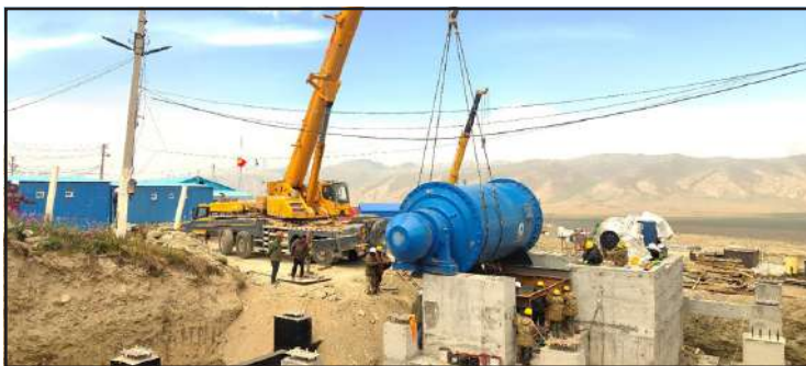
Figure 2 Installing the new ball mill.
