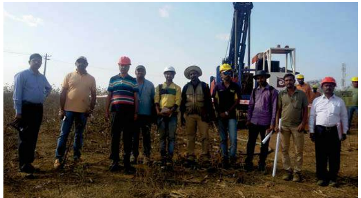
Fig-6:Diamond Core Drilling operation Ganajur Main Prospect
