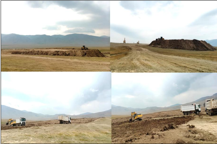
Figure 3: Excavation of the new tailings dam.
