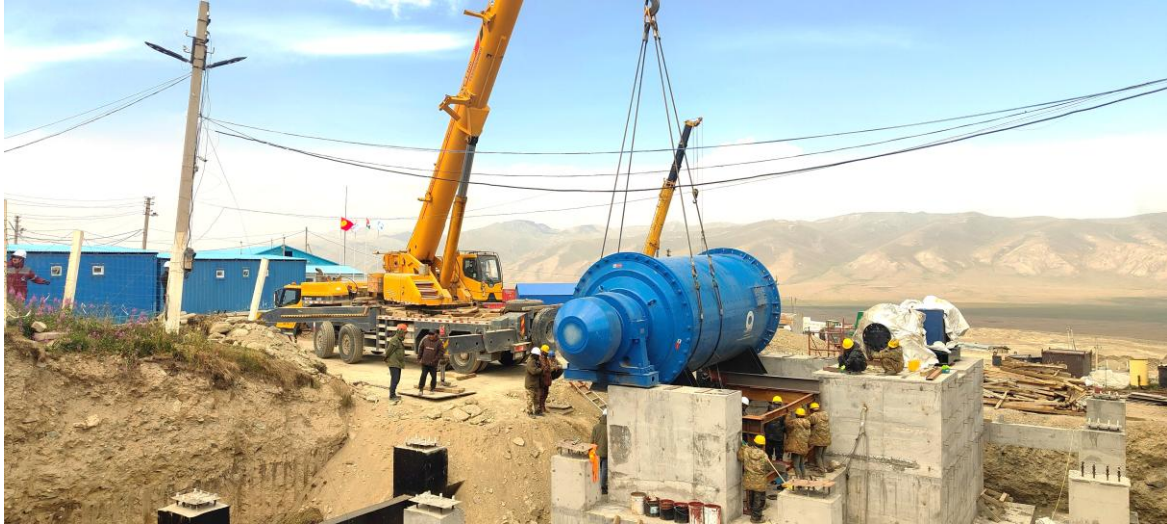
Figure 2: Installing the new ball mill.
